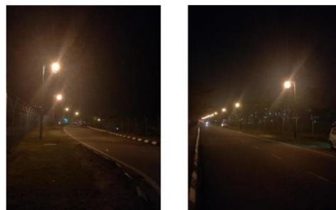
Figure 11. Active lamp posts at Mahallah Asiah on 29 March 2018
