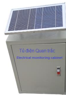
Figure 4. Monitoring cabinet (connecting sensors) meter for measuring water quality indicators
